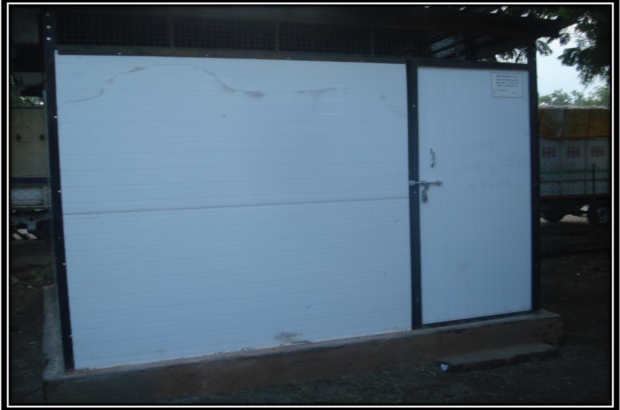
MDM: Kitchen shed under MDM
